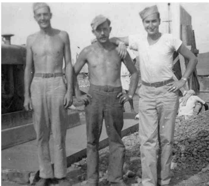
Three United States Army Air Force engineers standing in front of a water distilling pump and generator, probably India. (Image: The National WWII Museum, 2011.407.015.)
